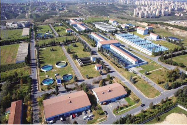
İkitelli Potable Water Treatment Plant
