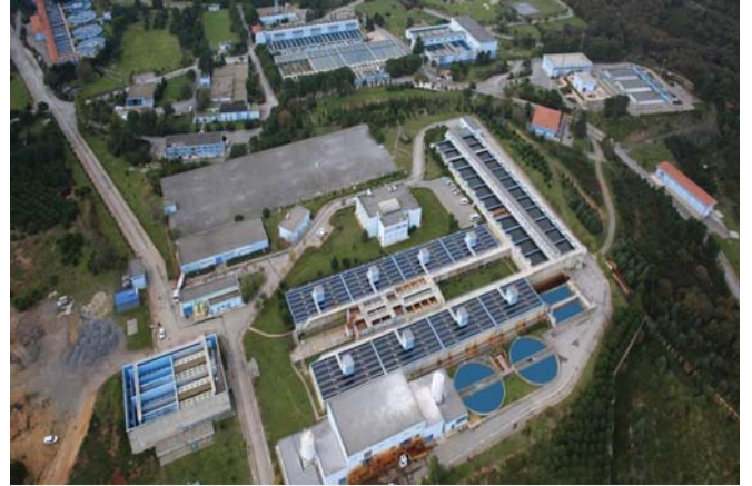
Ömerli Potable Water Treatment Plant
