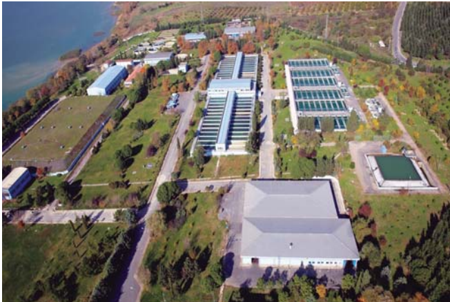
Büyükçekmece Potable Water Treatment Plant
