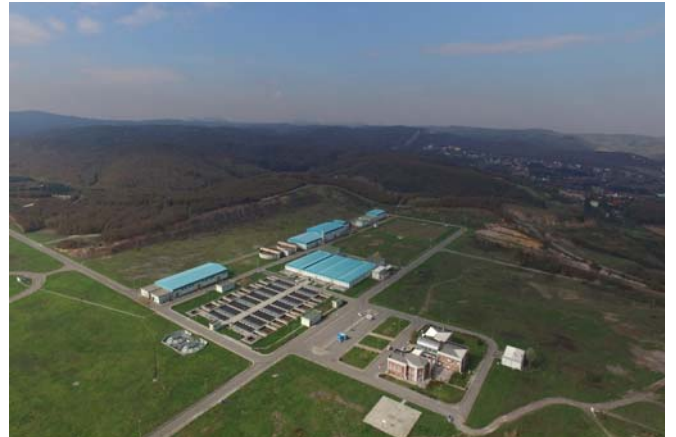
Cumhuriyet Potable Water Treatment Plant
