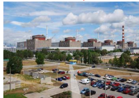
Zaporizhia Nuclear Power Plant (operations started in 1984-1987)
