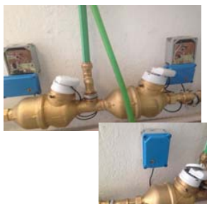
Smart meters deployment in OTE building at Ilissos for Smart Water Metering
