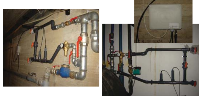
Sensor deployment in Main Supply and Student Residence for Water Quality Management
